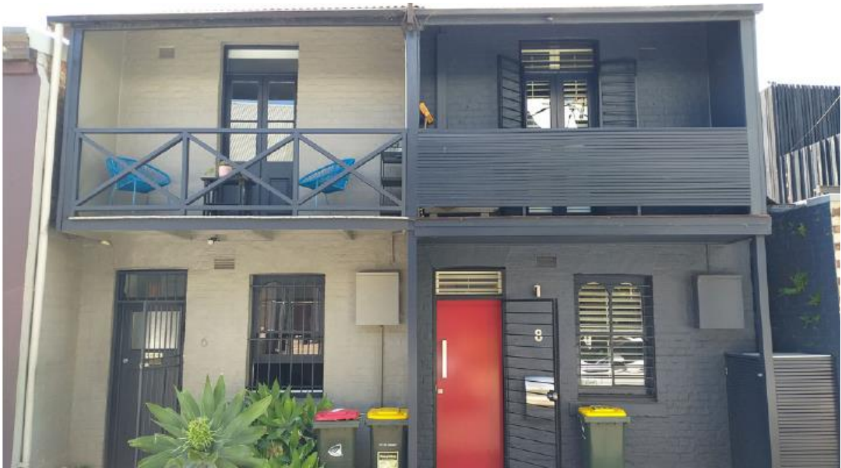
Figure 7: View of neighbouring terraces to the south (6 and 8 Raper Street)
