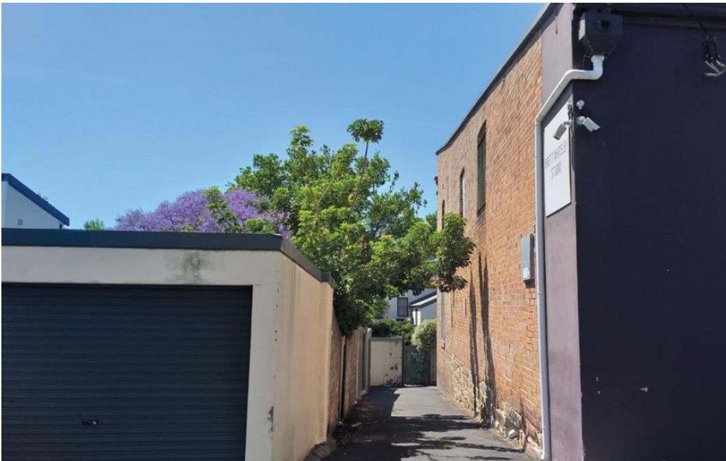
Figure 3: View of subject site to the north on Davies Lane
