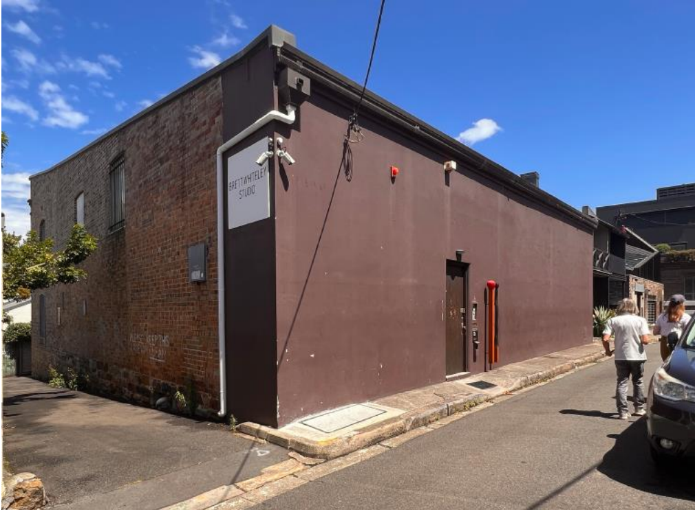
Figure 2: Site viewed from the corner of Raper Street and Davies Lane
