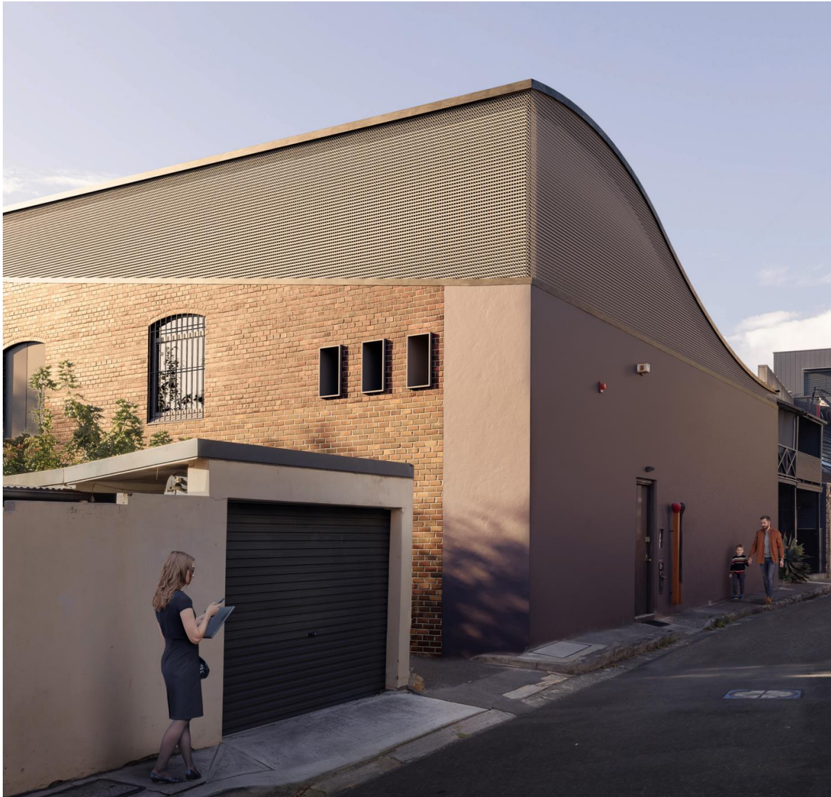
Figure 288: View of new windows on Northern Elevation
