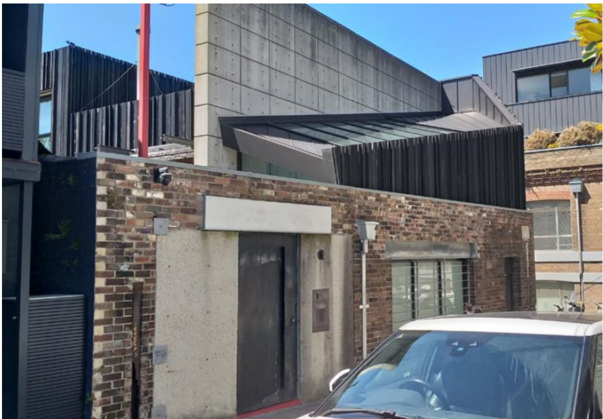
Figure 8: View of residential dwelling further south (1 Esther Street)
