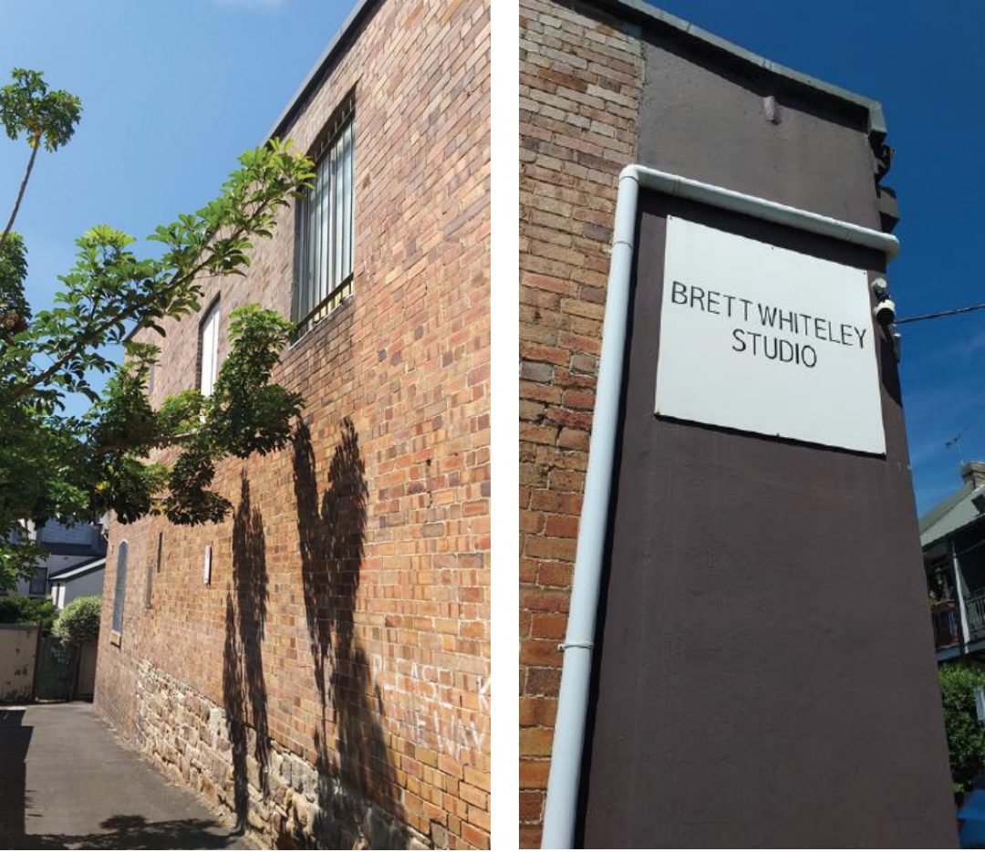
Figure 4: Existing northern elevation - windows and signage
